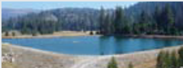
Bear Valley Water District Secondary Wastewater
