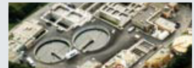
Sewer Authority Wastewater Treatment
